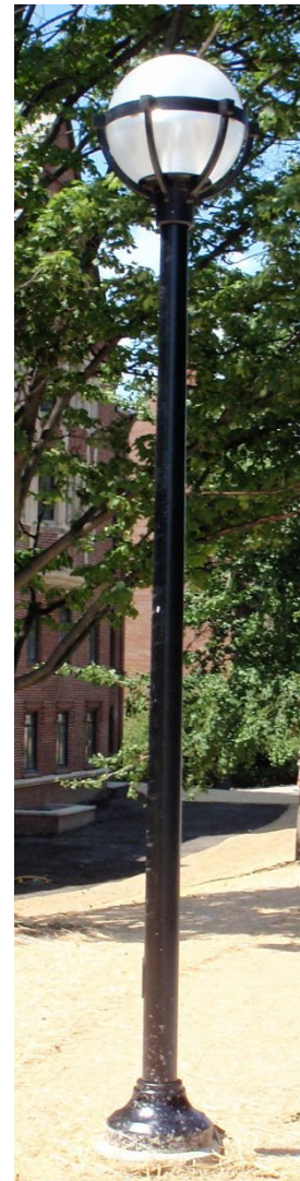
typical pedestrian scale light pole
