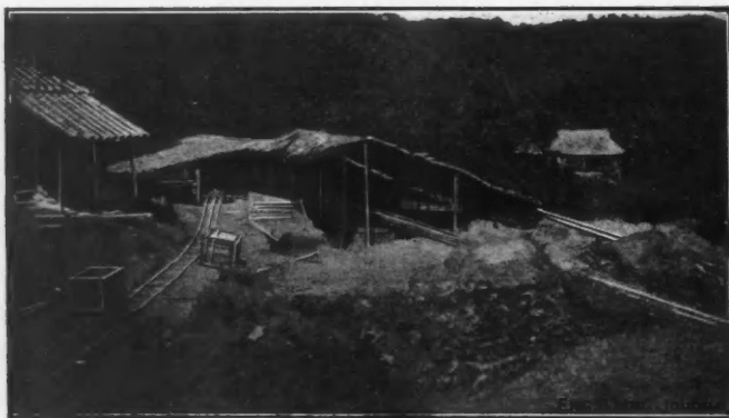
TWO TEMPORARY CYANIDE PLANTS IN COLOMBIA—NATIVE CANE PUMP RAISING CYANIDE SOLUTION
