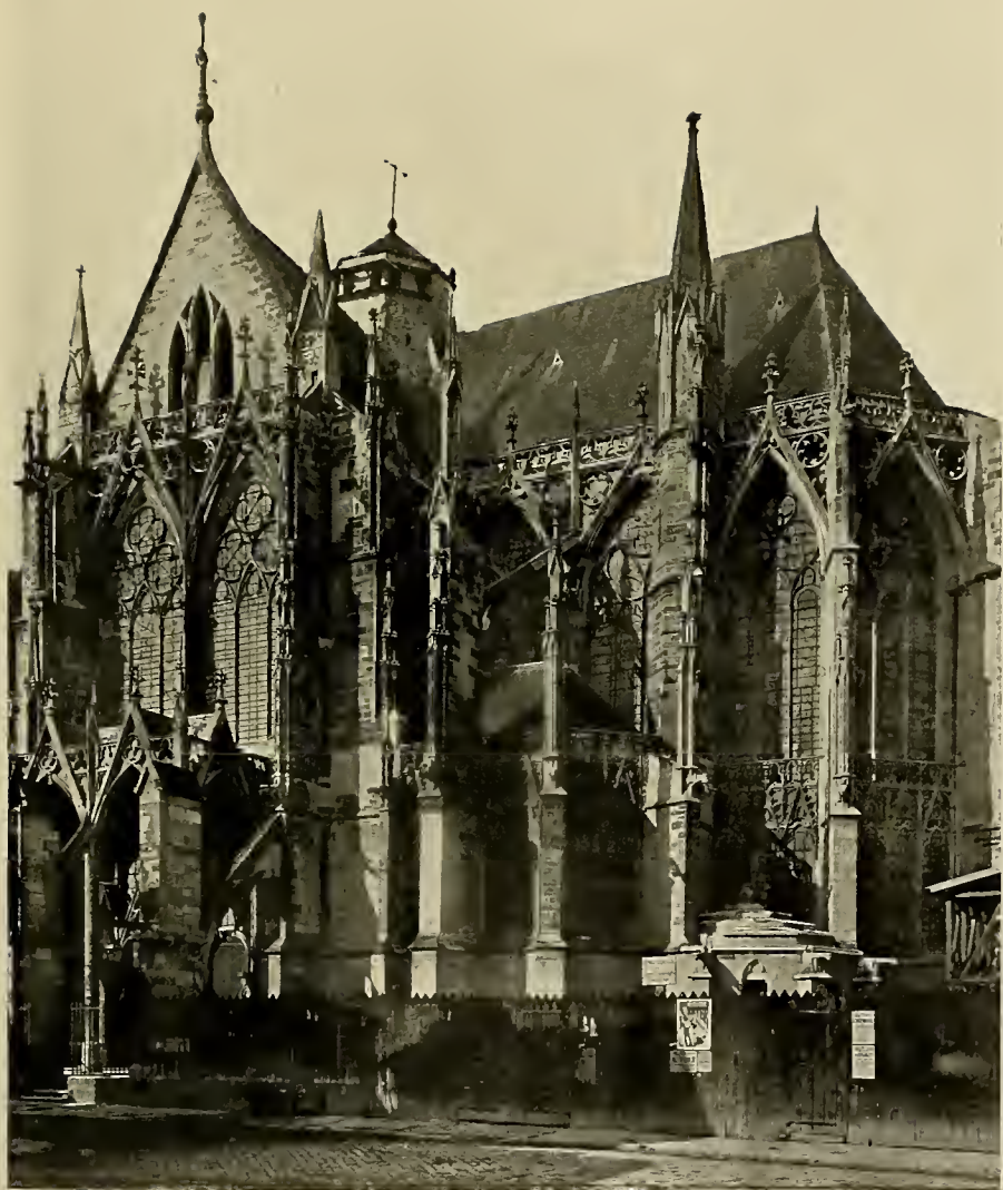
ILL. 220. — St. Urbain of Troyes, from the Southeast
