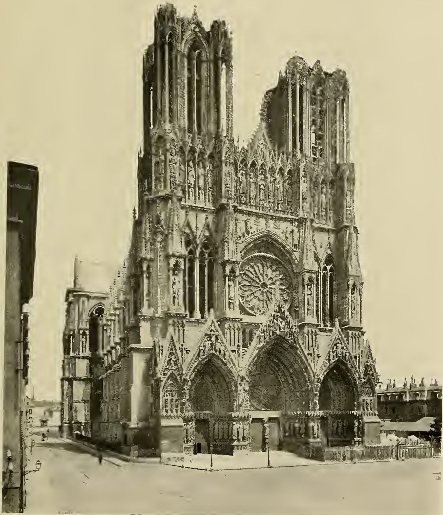
LI 224 — Façade of Reims
